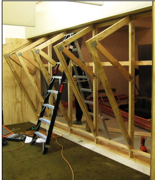
Figure 4: Installation of the trusses.
